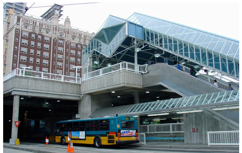
Seattle Bus Tunnel Convention Place Station
