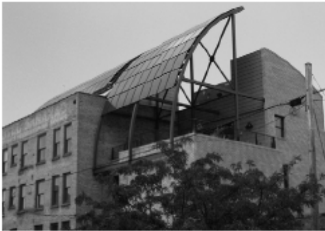
Spokane's Samac Building is one of only five LEED-platinum® certified structures in the State and the only one of its kind east of the Cascades. Originally a hotel built in 1908, the Samac now features a rooftop garden and a large solar panel array seen here that helped reduce building power consumption by 86%. (Washington State Department of Ecology)
