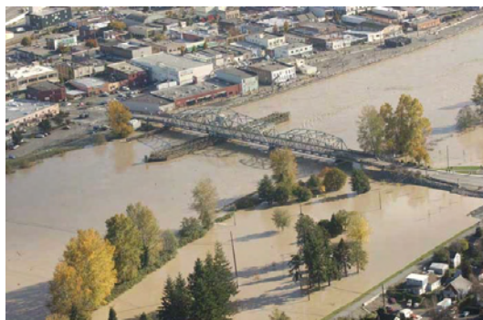
2003 Mt. Vernon Flood (Archive Photo, Skagit Valley Herald )
